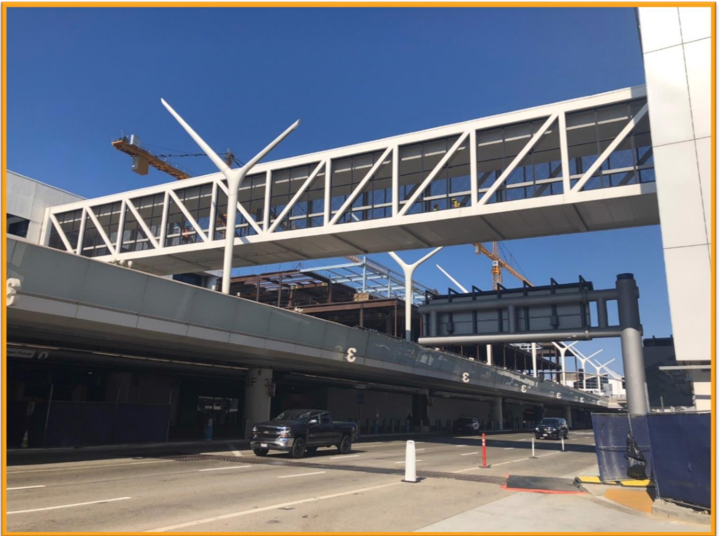
Terminal 3 / Parking Structure 3 Pedestrian Bridge to be demolished
