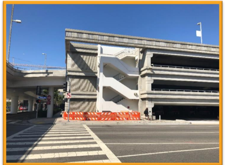
Parking Structure 1 APM Utility Investigations
