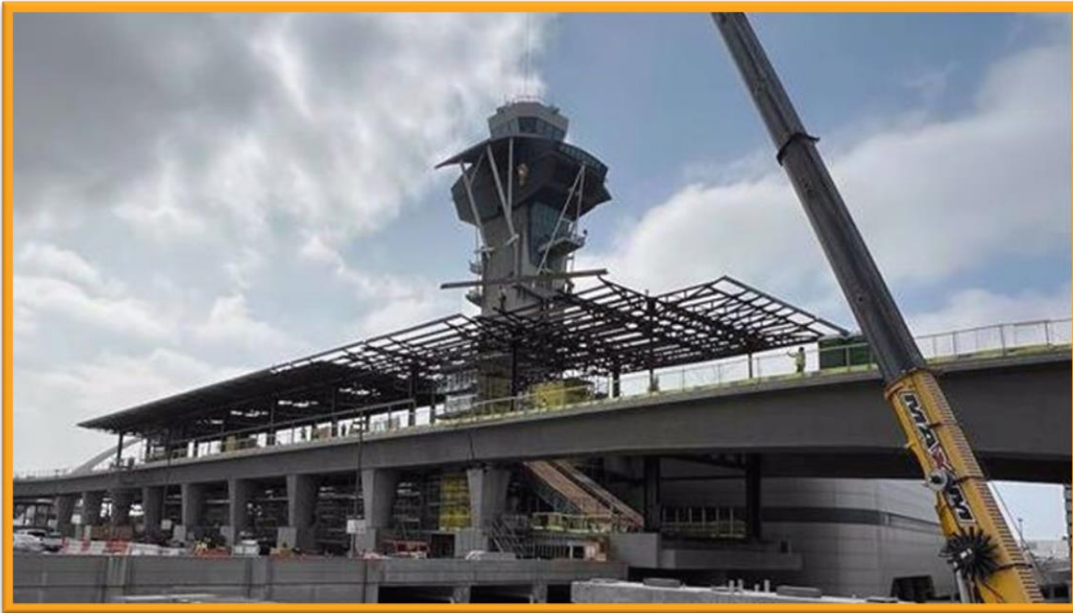
Left: Final steel placed at Center CTA APM Station
