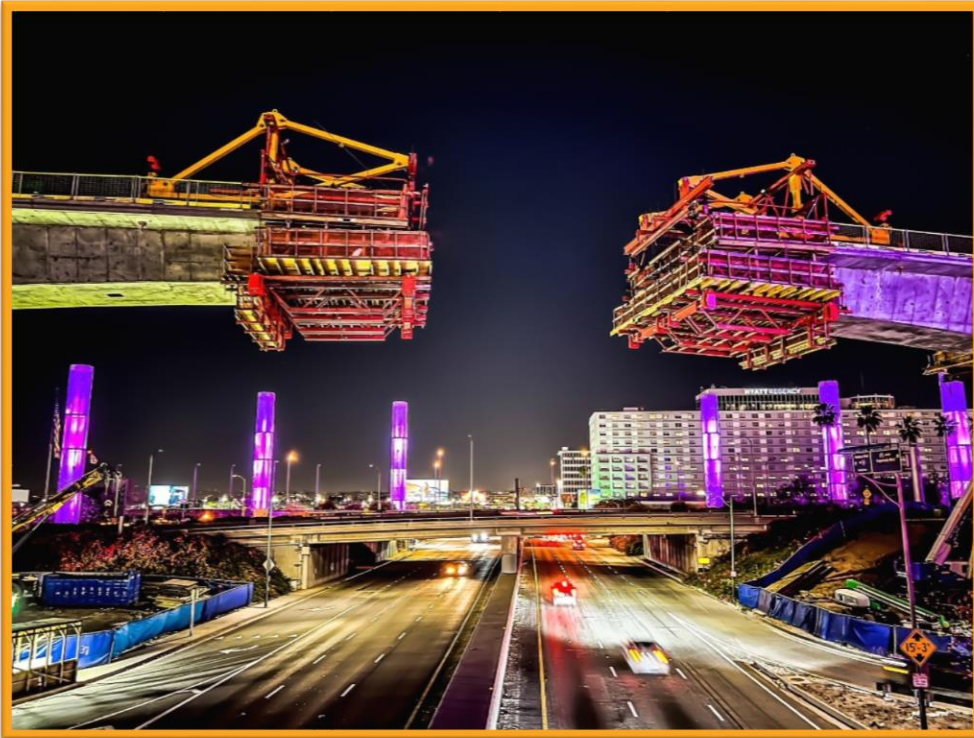
These two photos show APM guideway construction progress over Sepulveda Boulevard
