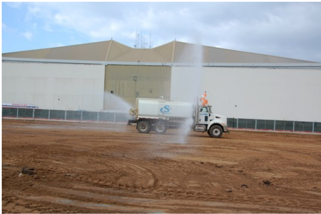
Figure 1.2.2-2: Dust Suppression Performed During Taxilane T Construction
