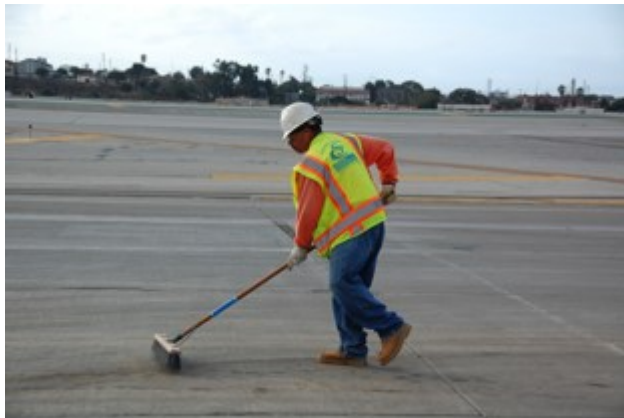
Figure 7-1: Dust Control Measures Being Implemented on Taxilane T
