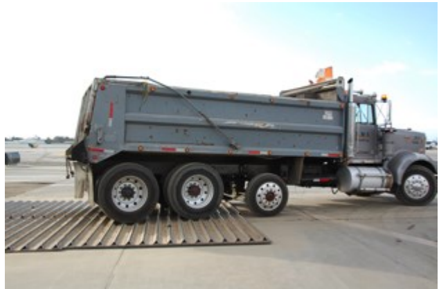
Figure 7-1: Dust Control Measures Being Implemented on Taxilane T
