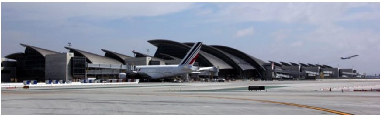
Figure 1.2.1-1: Tom Bradley Terminal Construction Progress as of December 2013
