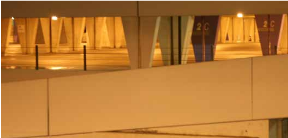
PARKING INTERIOR: HIGH PRESSURE SODIUM
