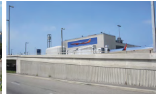
Terminal 1 - East Elevation
